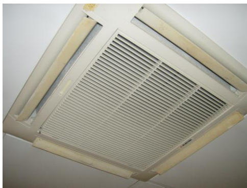
Fan-coil a soffitto
